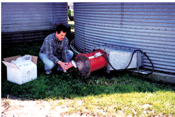
Figure 3. Aeration fan application
