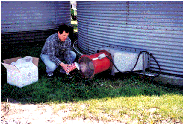
Figure 3. Aeration fan application
